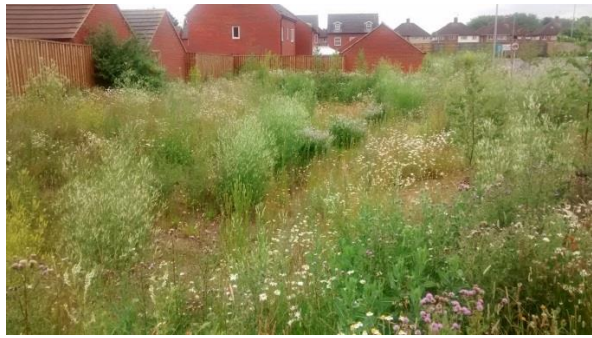
A new sustainable urban drainage scheme at a supermarket development
