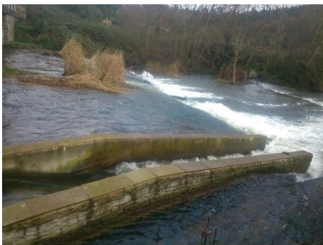
Fish and Eel passage at Lingen fish and eel pass on the River Teme.
